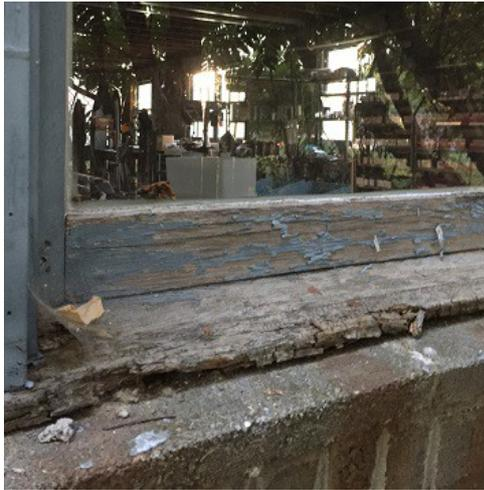
The next part of the project is the installation of new windows throughout the barn. On the first floor, the deteriorated wood sash and frame windows will be replaced with custom vinyl-sided, single-hung windows. Benefits will include improved ventilation, better security, increased property value, and overall enhanced appearance.
